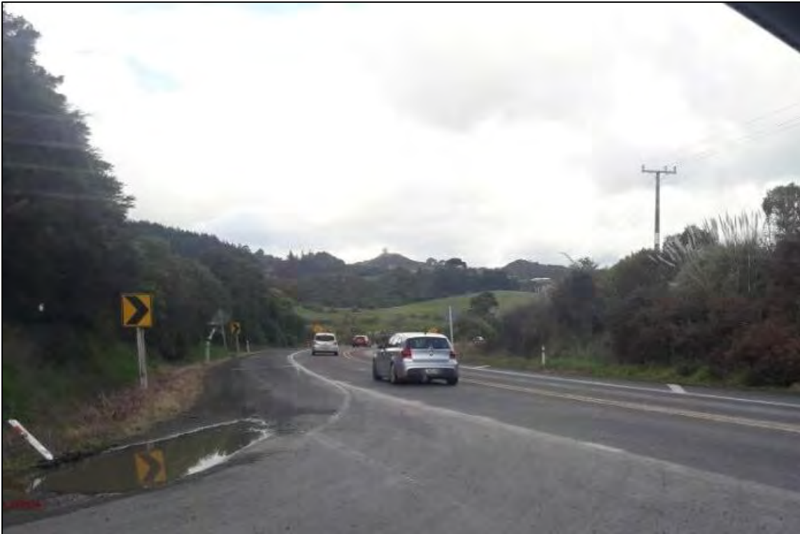
Figure 8: Existing ponding at the SH2/McPherson Road intersection and faded limit line markings.
