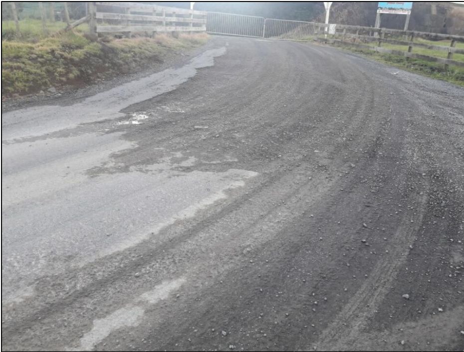
Figure 5: Existing vehicle crossing and poor condition of surface
