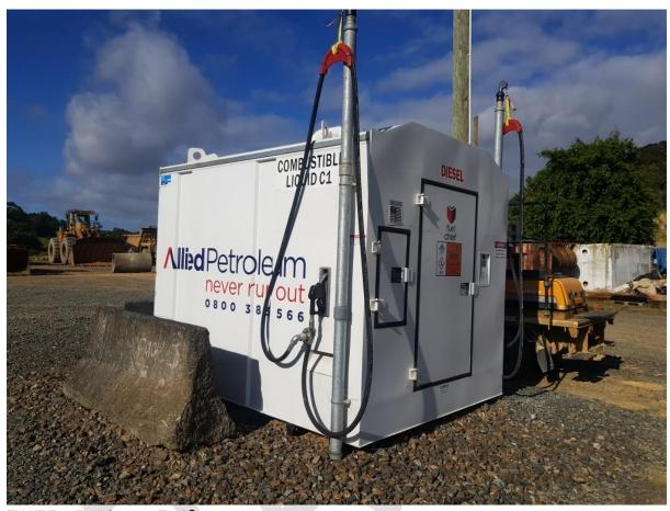
FIGURE 1: Fuel Storage Tank<sup>7</sup>
